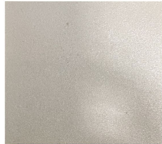
Spiral Stair Case Surround Plaster
